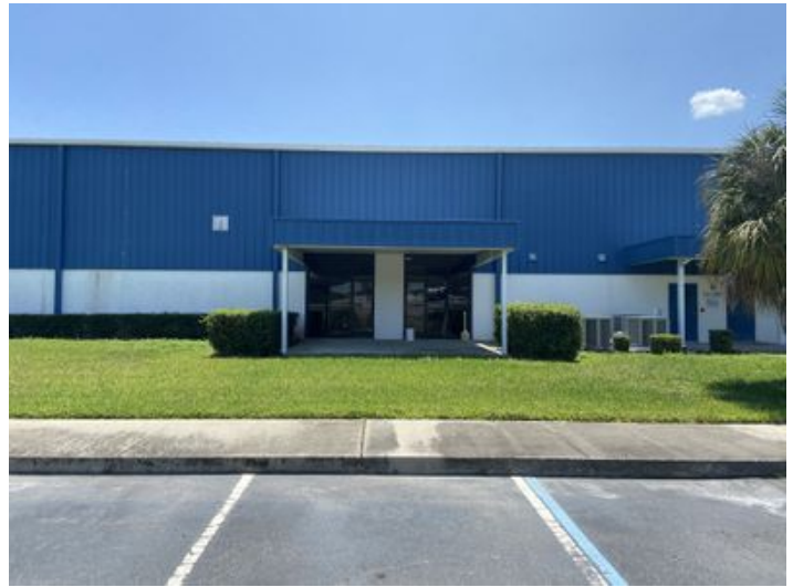
Employee Entrance-Exit to Parking Lot
