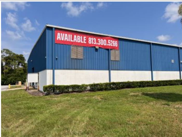
Building Facing I-275
