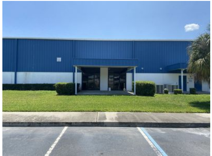
Employee Entrance-Exit to Parking Lot
