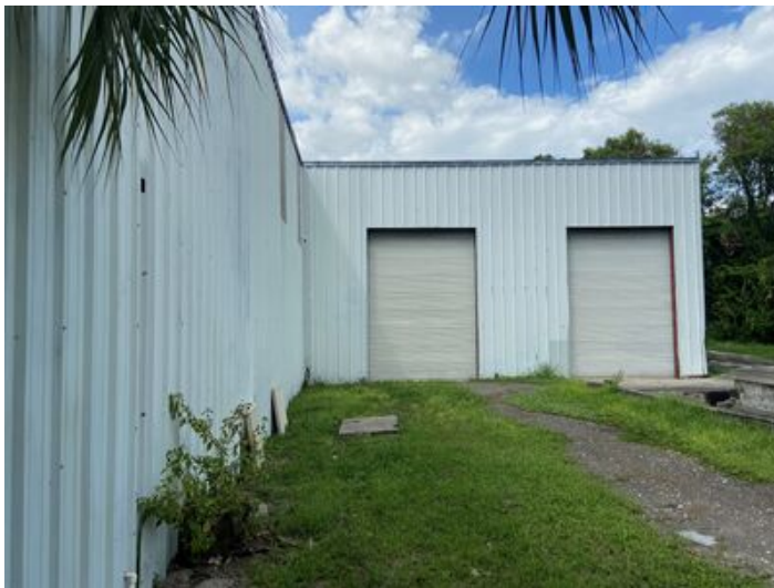
10' x 14' Loading Doors (Dock Well + Grade)
